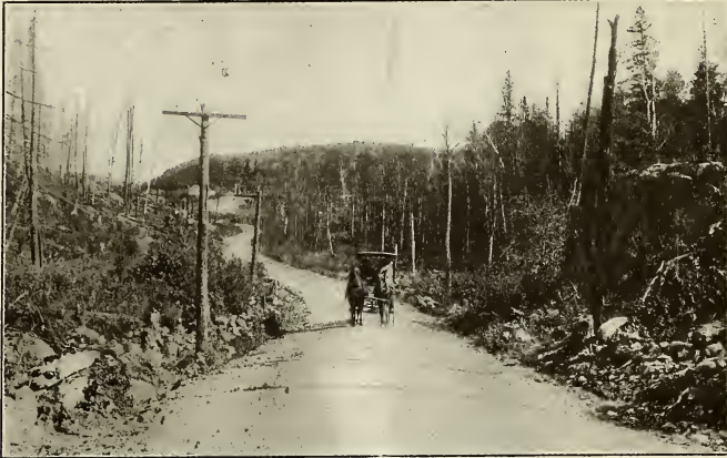
A GOOD ROADWAY OVER THE ROCKS NEAR COBALT
